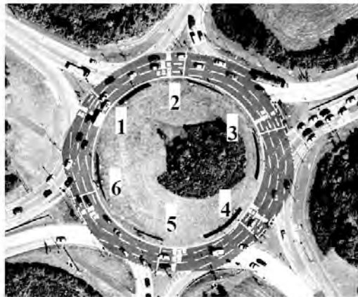
Figure 1. The Sheriffhall Roundabout. Source: Google Earth.
